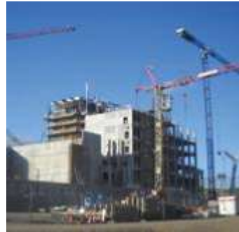
Filborna Power Plant Sweden 2011-2012 PLN 26.2 million
