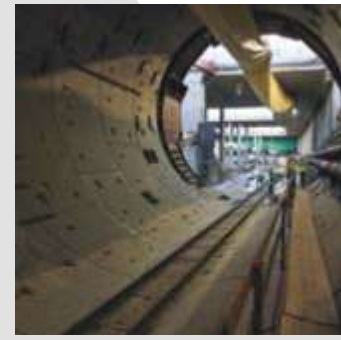
Tunnel under the Martwa Wisła river Gdańsk 2013-2014 PLN 44.9 million
