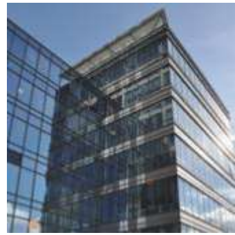
Olivia Business Center Gdańsk 2010-present PLN 144 million
