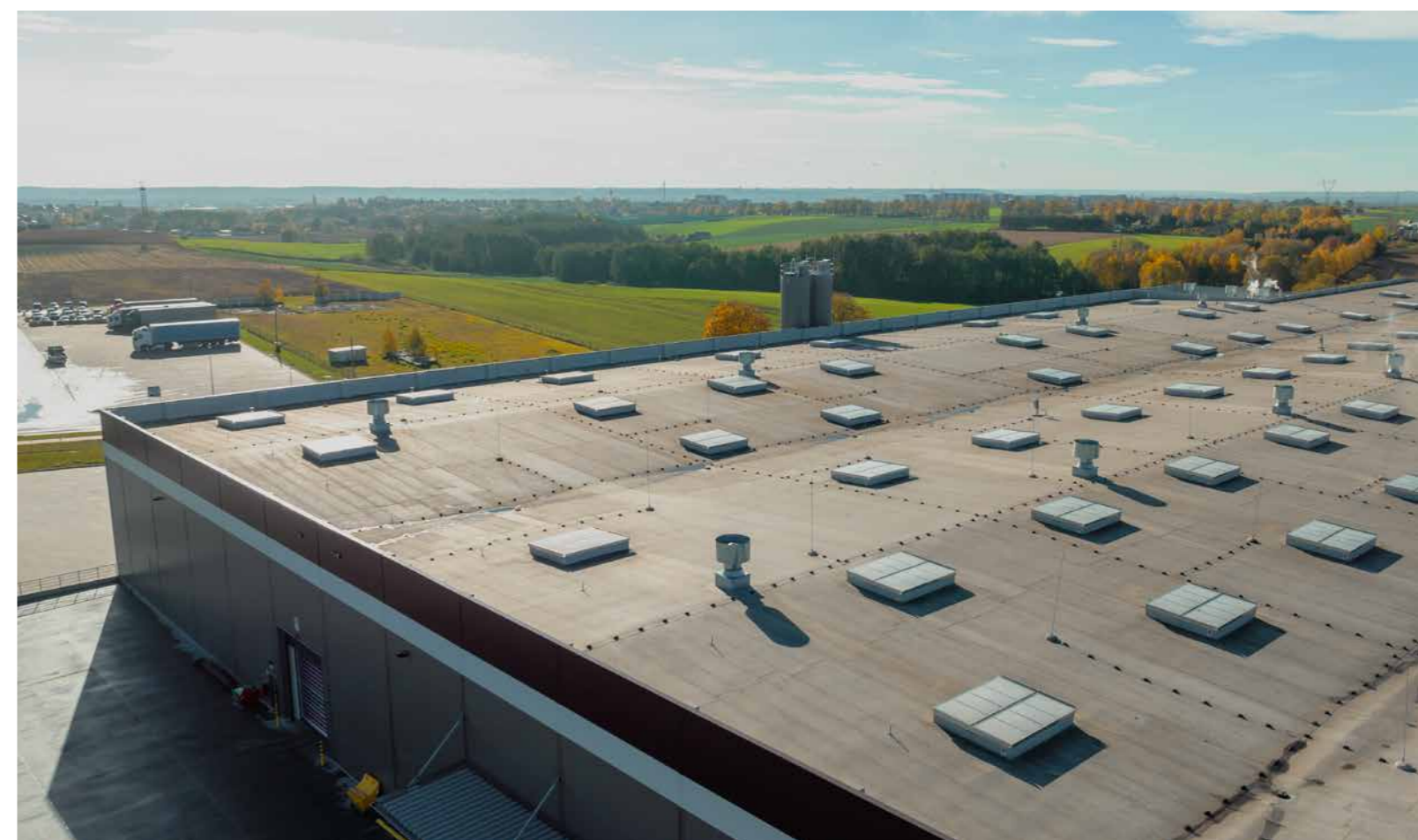
Hala Bart, Sulnowo
