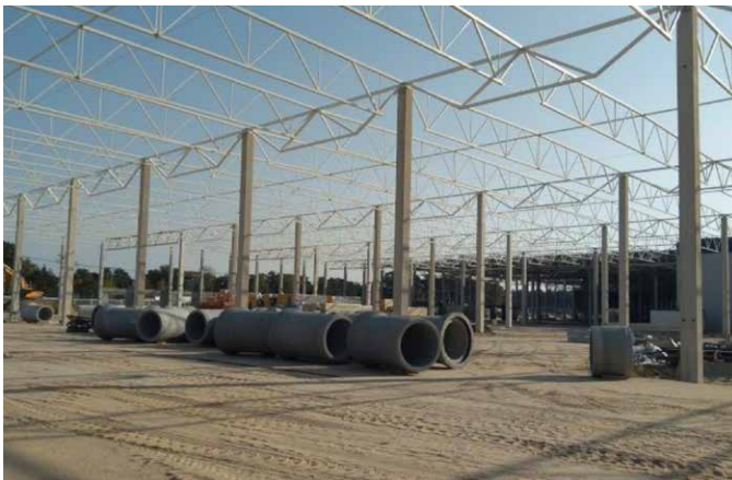
Photo 3. Roof of the hall made using steel prefabrication technology [S5].
