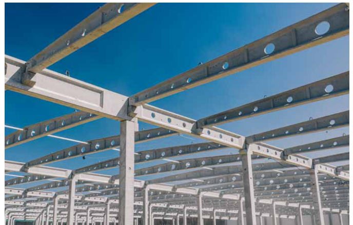
Photo 4. Roof of the hall made in prefabricated prestressed concrete technology [PEKABEX].
