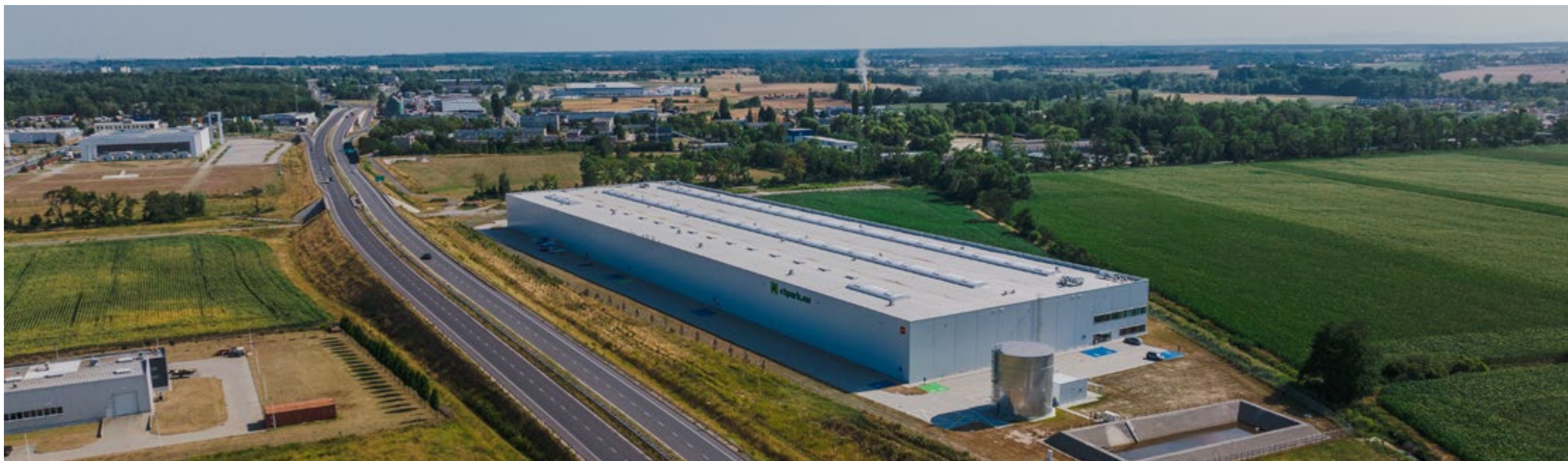
CTPark hall, Opole
