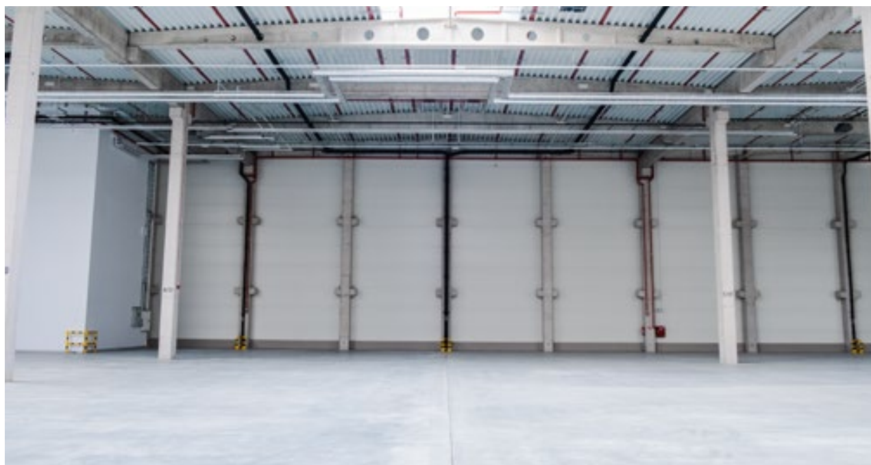
CTPark hall, Opole
