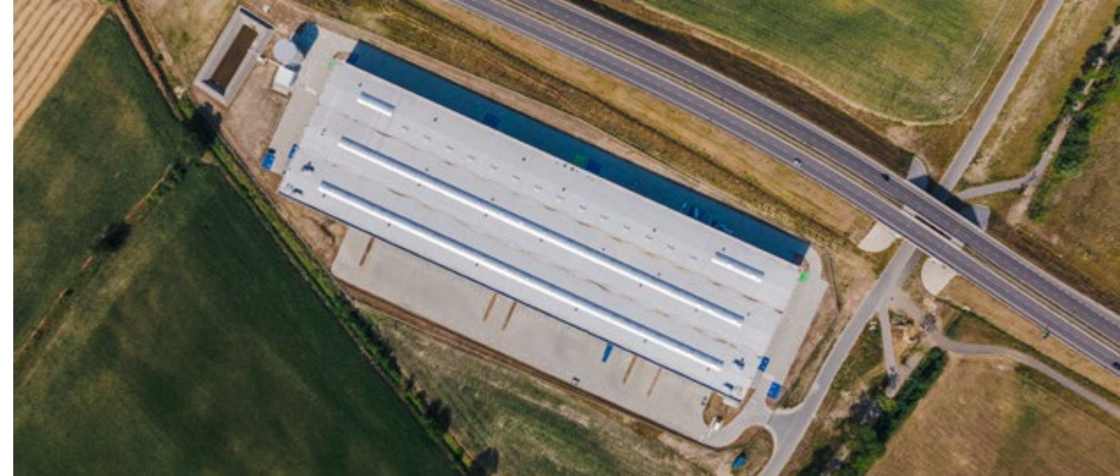
CTPark hall, Opole
