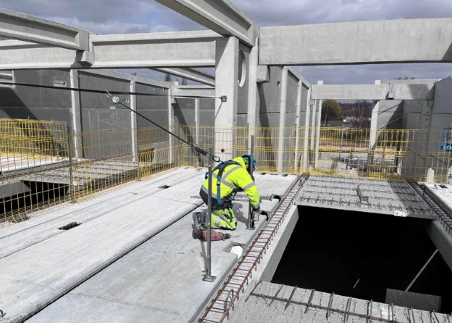
Assembly worker on the construction site
