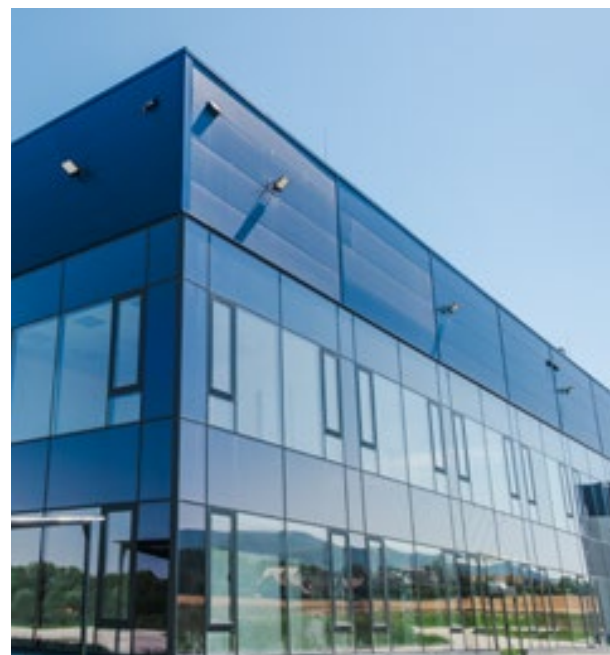
Social and office facilities, Panattoni Park III hall, Bielsko-Biala
