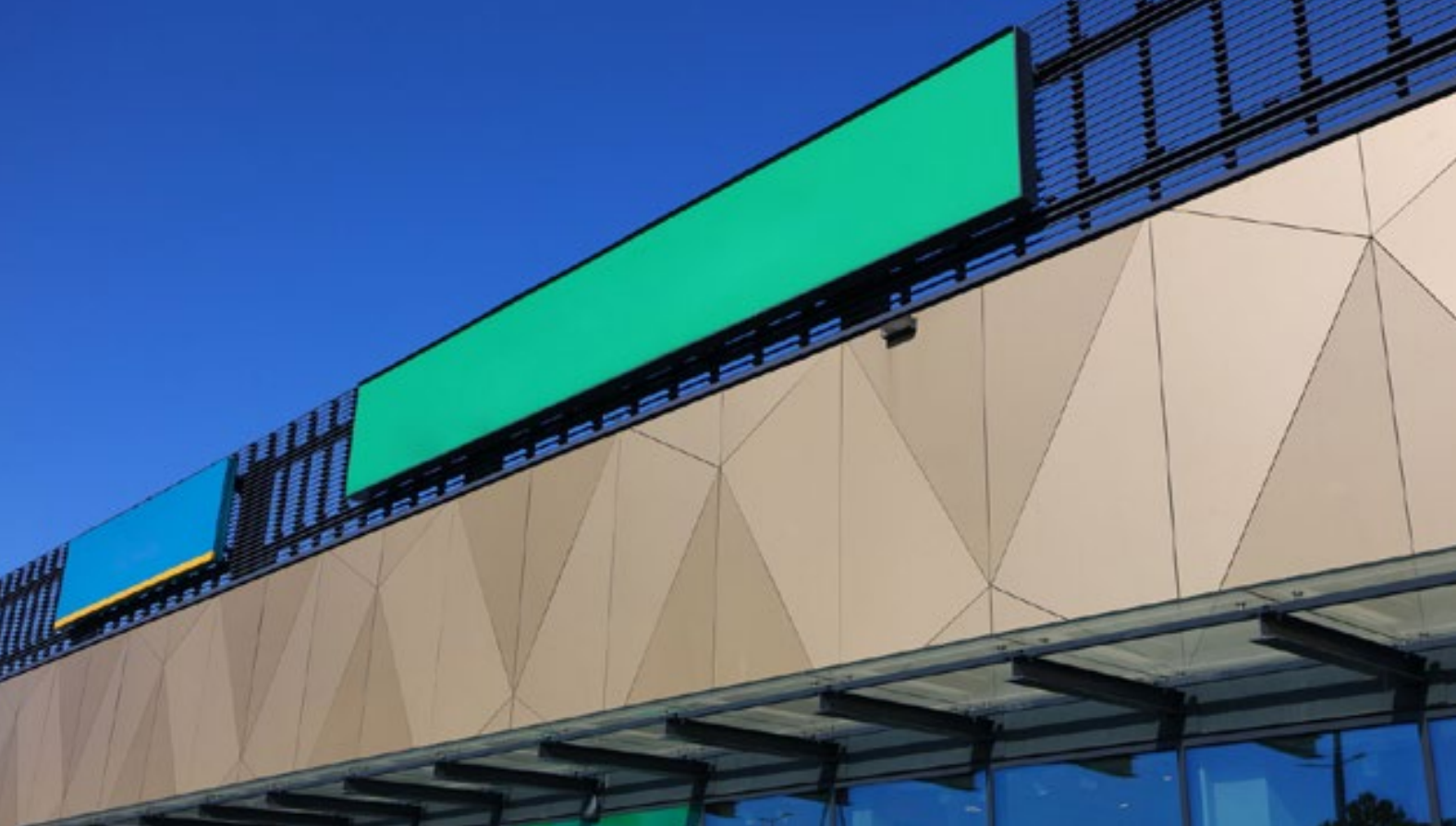
Retail facility for Budner, Piastów
