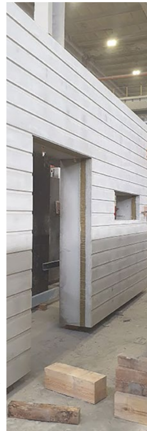
Prefabricated three-layer wall, Pekabex Gdańsk
