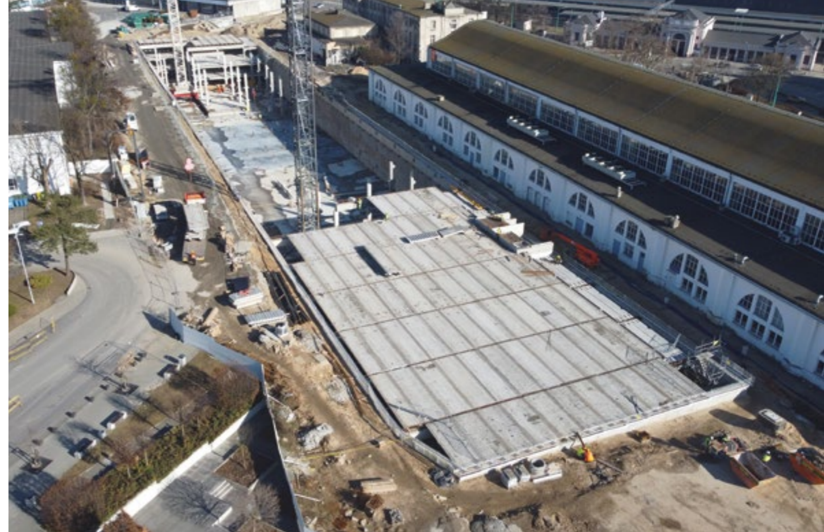
Underground car park, Poznań International Fair, Poznań
