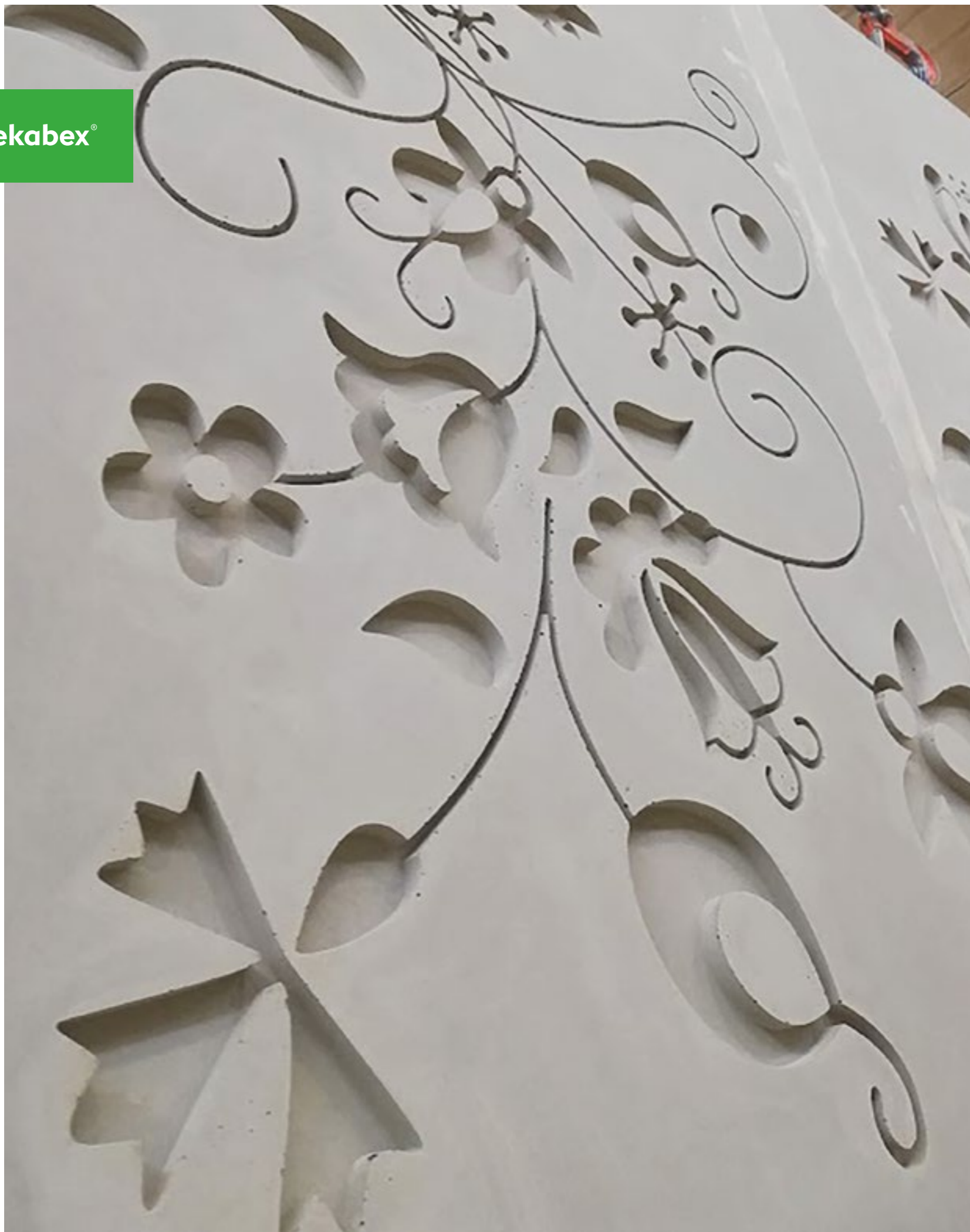
Prefabricated wall with matrix, Pekabex Gdańsk
