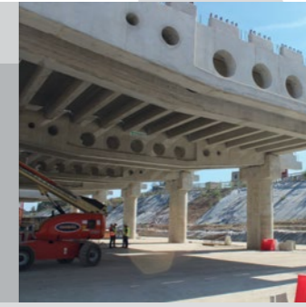
Łódź Fabryczna railway station 2014-2016 PLN 43.7 million
